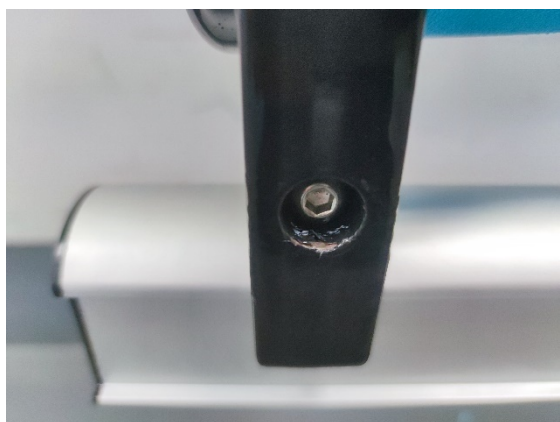
After 240 hours test - View 9
